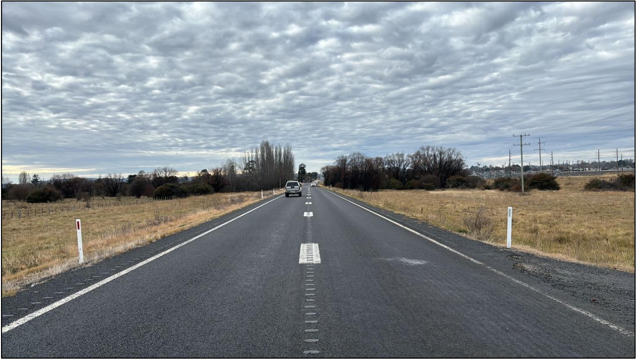
Figure 4: Gwydir Highway eastbound, adjacent to the subject site (to the right)
